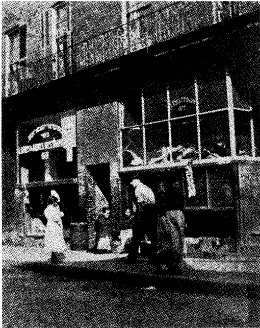
A Kosher restaurant in the North End
