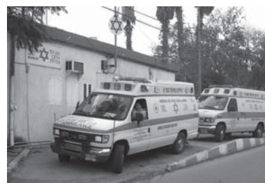
The current MDA Station in Sderot is a single level structure built in the 1950s. It is outdated and in such poor condition that the municipality has declared it a hazard.
