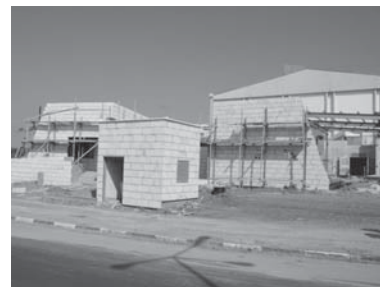
New Sderot Station is nearing completion
